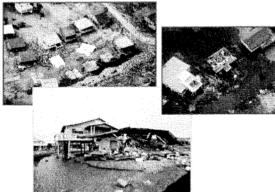
Damage left behind from Hurricane Ike. Photos courtesy of Dan Dalstra, The Facts.
